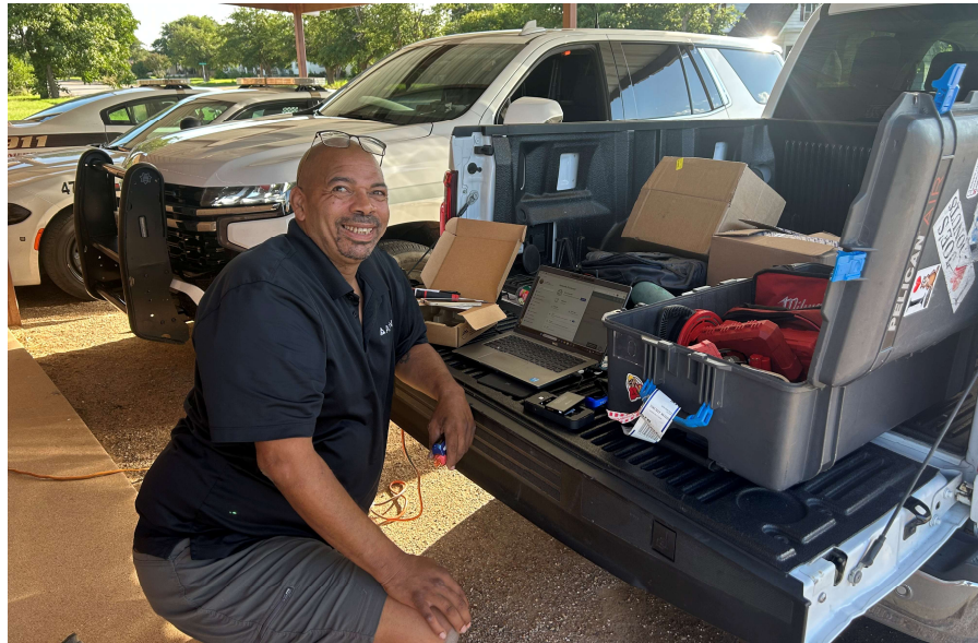
Pictured above is AXON Representative Larry Thomsen installing the new ALPR Cameras into the City of Seymour Police Cars.
