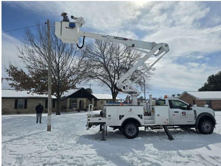
Pictured above, Electric Department employee Johnathon Olinger works from the bucket repairing a connection in frigid temperatures, while Gareth Hons stands below monitoring the area to ensure safety.
