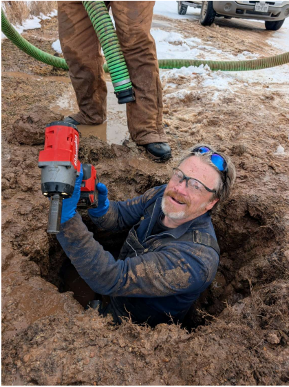
Jay Smith, pictured above, works neck deep in frigid conditions repairing a water leak with assistance from the Water Department, demonstrating dedication to keeping city services running.
