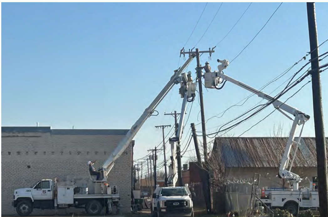
Pictured above Electric Department team consisting of John Joyce, Garet Hons, and Jonathan Olinger replace a bad transformer on Monday.
